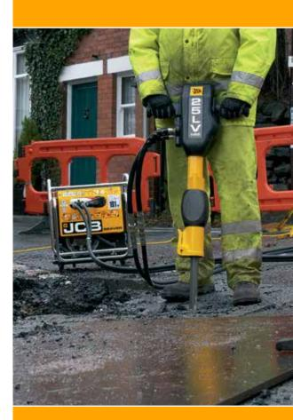
New ultra low vibration system: reduces hand arm vibration by 60% to 1.6m/s² (single axis)
