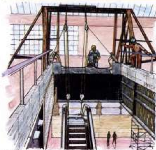
Fig. 28 - Installation of mechanical escalator (TU-26H)
