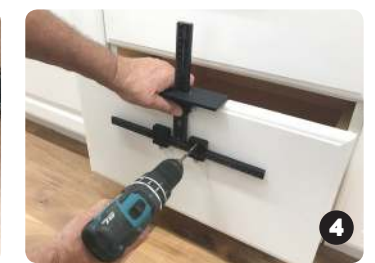
Center on drawer and drill holes
