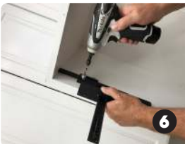
Drill top hinge holes
