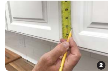
Measure from bottom mark position with pencil
