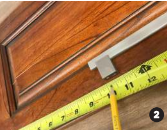
Measure from left of drawer to center of left hole on hardware. Use half this to set for the sliding stop end on the era
