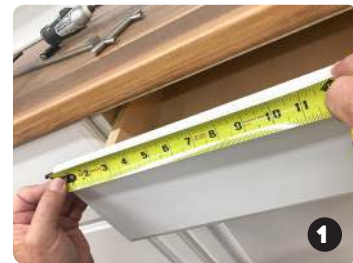
Measure width to find center
