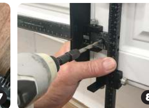
Position tool as shown drill through fixed center bushing for bottom hole
