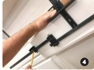
Set small end stop to half the drawer width
